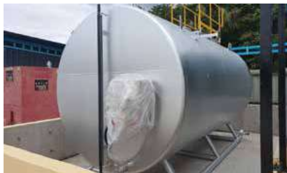
Aboveground Fuel Tank with UL 142 Listed (Double Wall / Single Wall)
