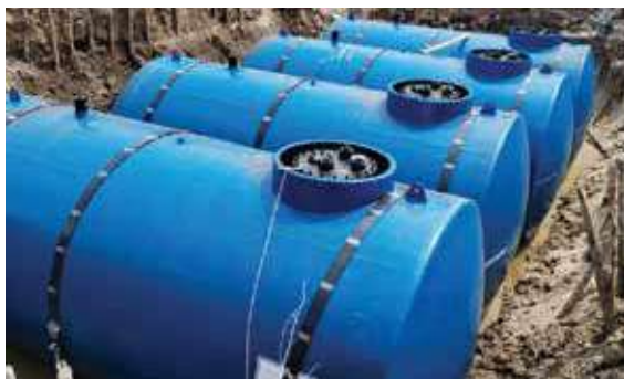
Underground Fuel Tank with UL 58 & UL 1746 Listed (Double Wall / Single Wall)
